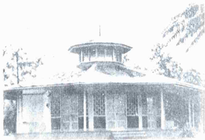
Fig. 55. The old Surau built in 1960, had been demolished to give way to the Tun Haji Ahmad Zaidi Adruce Auditorium. A new Surau is being built behind the Men's Hostels at the time of writing. Photo: Mr. Lim Yu Seng
