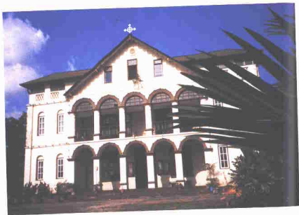
Fig. 11 The Catholic Centre, Built in 1913, along Tun Hj Openg Road near to St. Teresa's Secondary School Hall, used as the Japanese Court House during the War. Photo: Mr. Fong Hon Kah
